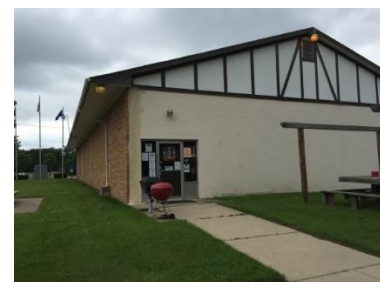
POST 2645 entrance in the rear of the building
